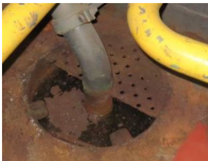
LHD well deck grating*
