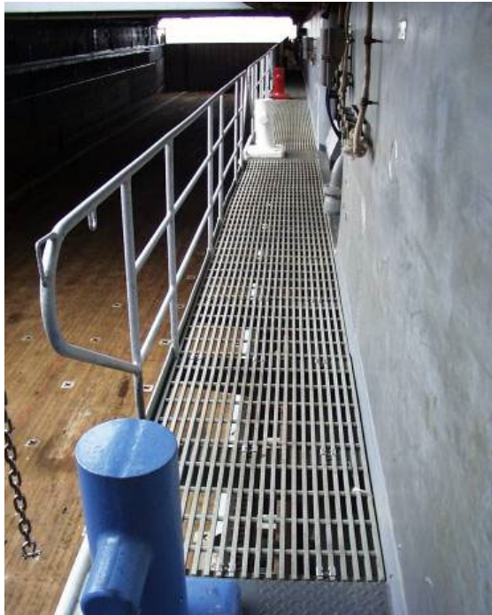
LSD Wing Wall
