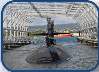
Magnetic Silencing Deperm Facility (Beckoning Point, PH)
