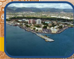
Submarine CSI Support (SUBBASE, PH)
