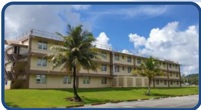
• Shipboard Electronic Systems Evaluation Facility (SESEF)
