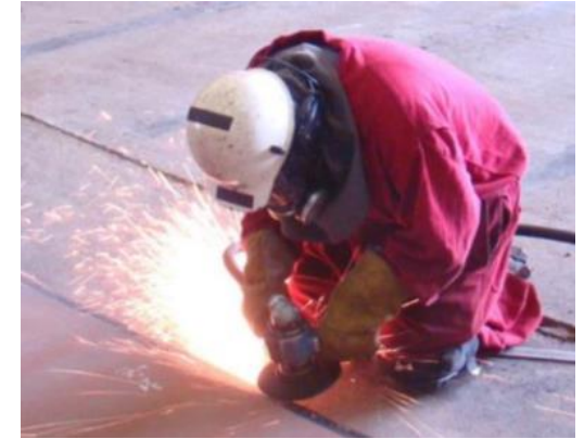
Manual grinding removal of PCP
