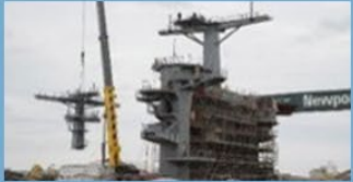
Aircraft Carrier Refuelings (RCOH) & Inactivation
