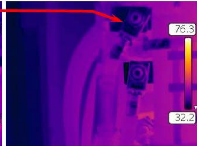
After Repairs Thermogram
