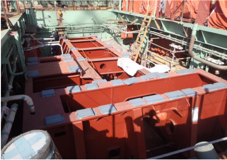
Main Engine Foundation
