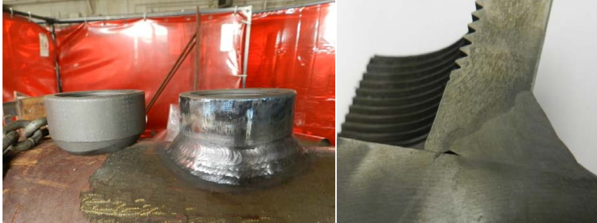
Figure 15 – Carbon Steel Boss Weld
